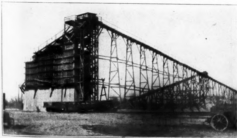
View of Storage Plant Taken Just After Completion
